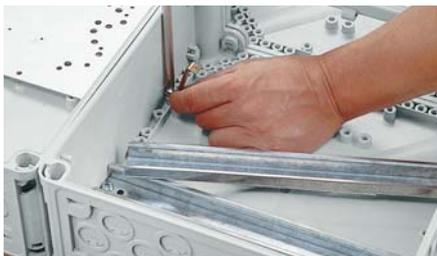
■ Equipment can be installed via DIN rails which are fastened on spacers
