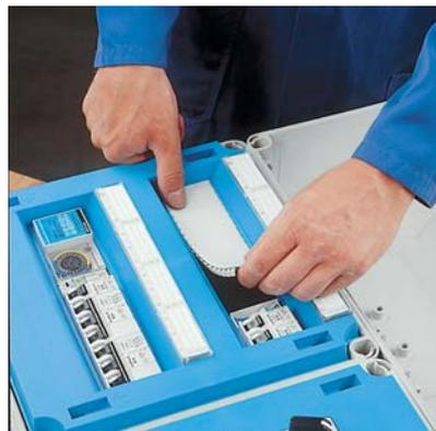
**Device installation in circuit breaker boxes**
